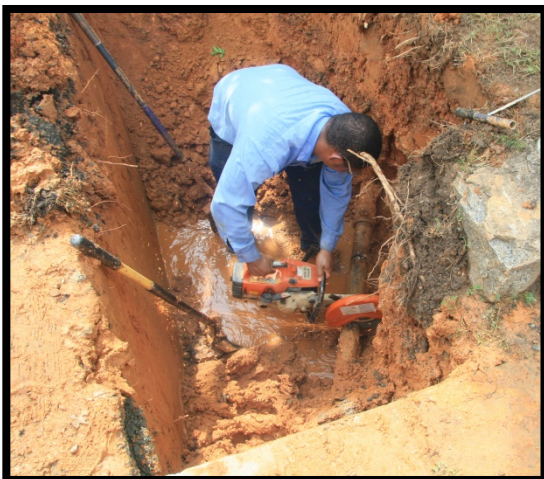
Pictured: Roger Smith repairing a water pipeline
