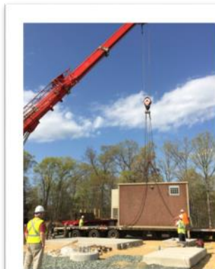
A crane is used to place the shelter at the Columbia School site.
