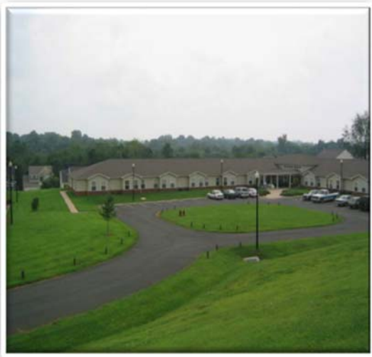
MOUNTAIN RUN Culpeper, VA Completed: 1999 50 Senior and Family Affordable Apartments Total Development Cost: $3 million
