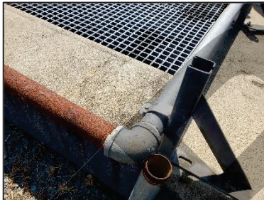
Figure 87 - Rusted Pipe
