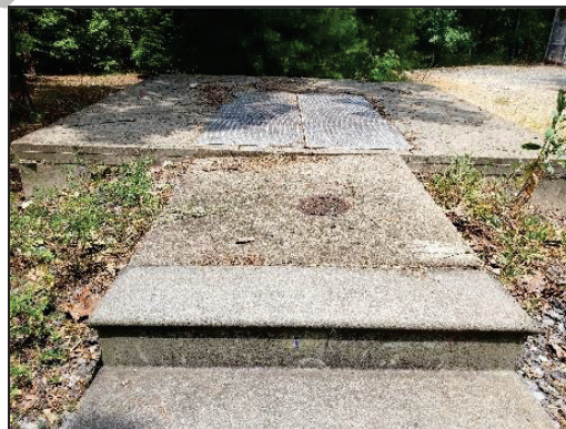
Figure 44 - Valve Vault Exterior
