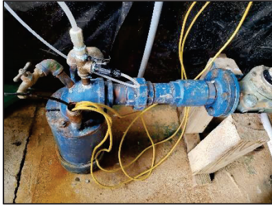
Figure 70 - Loose Wiring
