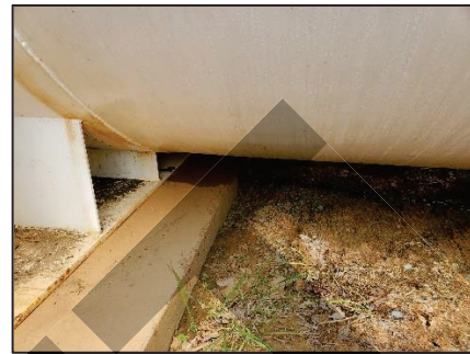
Figure 3 - Backwash Tank Support
