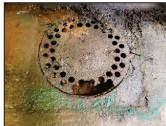
Figure 51 - Broken Drain Cover
