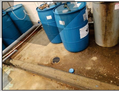
Figure 11 - Chem System Containment
