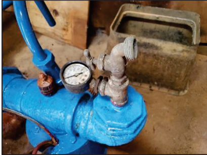
Figure 15 – Threaded Sample Tap
