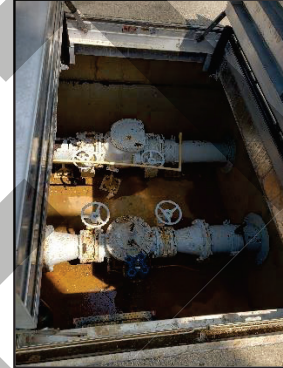
Figure 37 - Valve Vault
