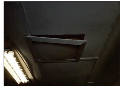
Figure 31 - Damaged Ceiling
