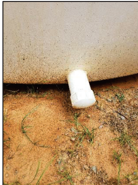
Figure 2 - Backwash Tank Drain
