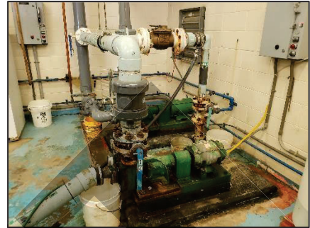
Figure 23 - Buckets Where Pipes are Leaking
