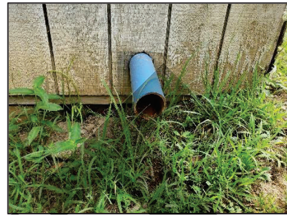
Figure 20 - Well House Blow Off
