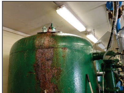
Figure 13 - Tank Manway Rust
