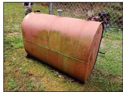
Figure 6 - Diesel Storage Tank
