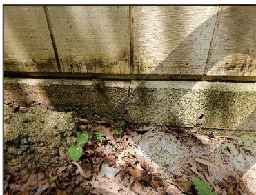
Figure 45 - Concrete Base Cracks
