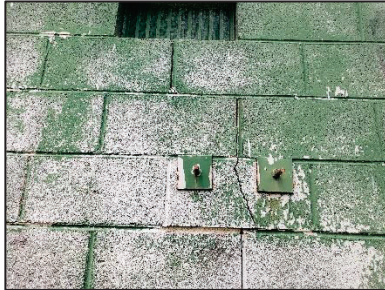
Figure 35 – Damaged Blockwork
