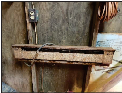
Figure 1 – Well House Heater
