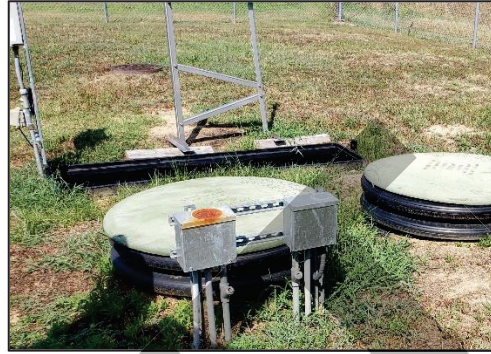
Figure 79 - Rusty Junction Box
