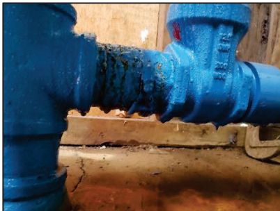
Figure 18 – Well House Leaky Piping
