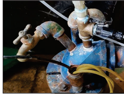
Figure 71 - Threaded Sample Tap
