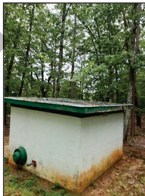
Figure 53 - Tin Roof Rust
