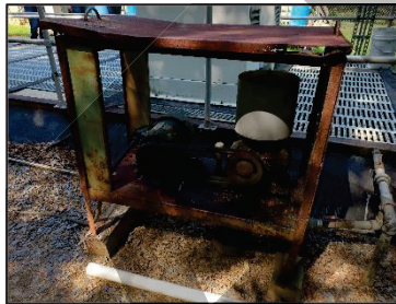
Figure 84 - Blower and Housing
