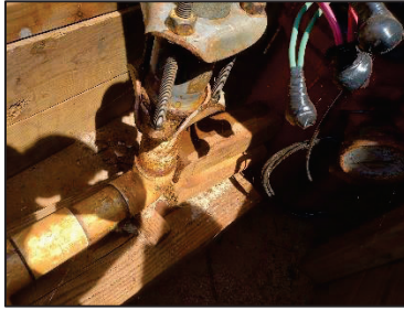
Figure 41 - Well Pump Bracing
