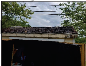
Figure 65 - Roof Shingle Peeling
