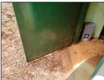
Figure 55 - Rotting Door
