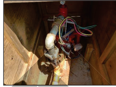
Figure 42 - Loose Wires in Well Housing
