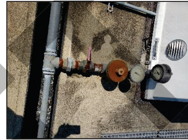
Figure 92 - Air Release Valve
