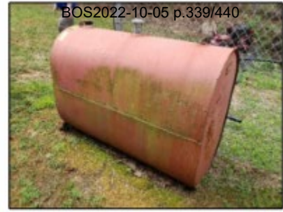
Figure 6 - Diesel Storage Tank
