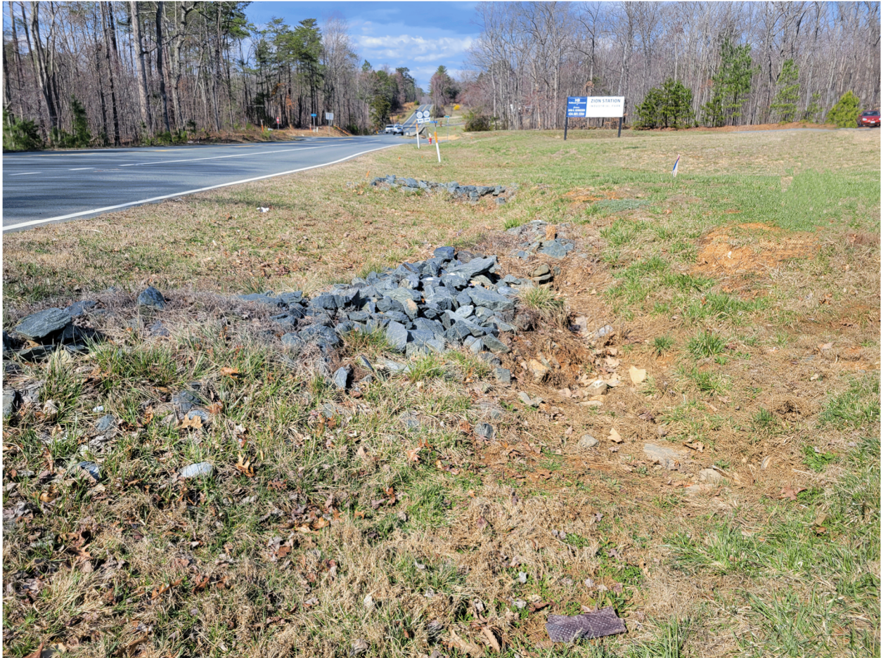
Site Photo 2 – Basin Discharge and Downstream Ditch
