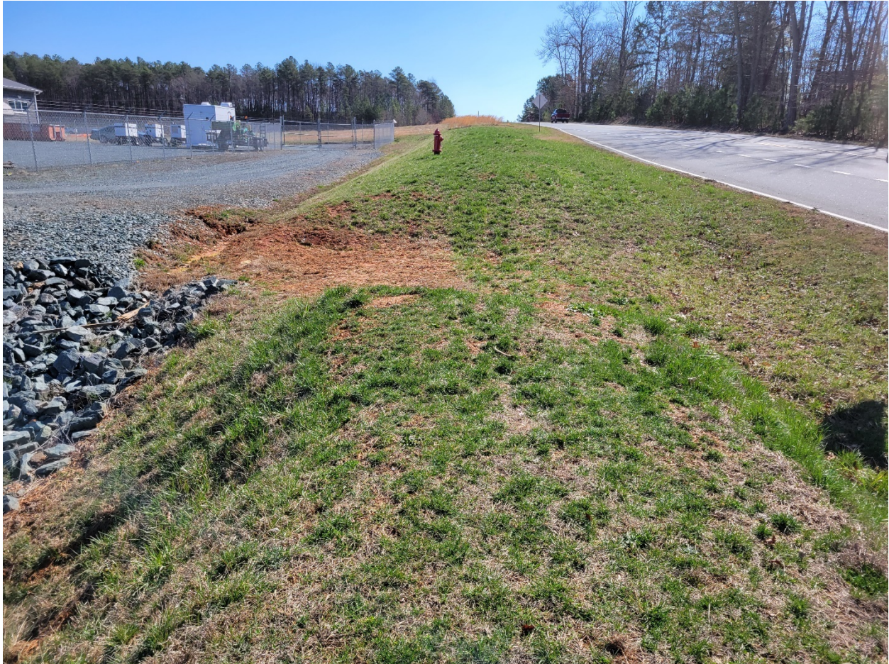
Site Photo 1- Ditch and Emergency Spillway.
