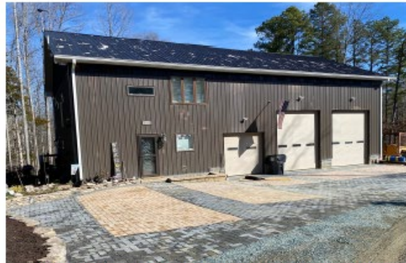
Fluvanna County resident, Eric Shrieves, was awarded funding by VCAP to implement a permeable pavement project on his property.
