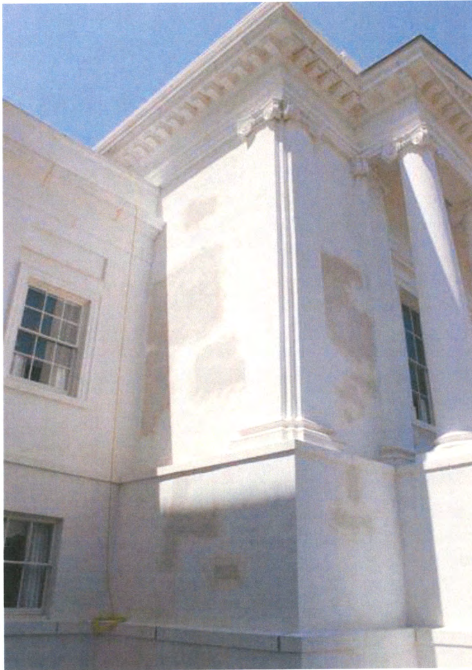
Figure 3: Virginia State Capitol, Stucco Repairs
