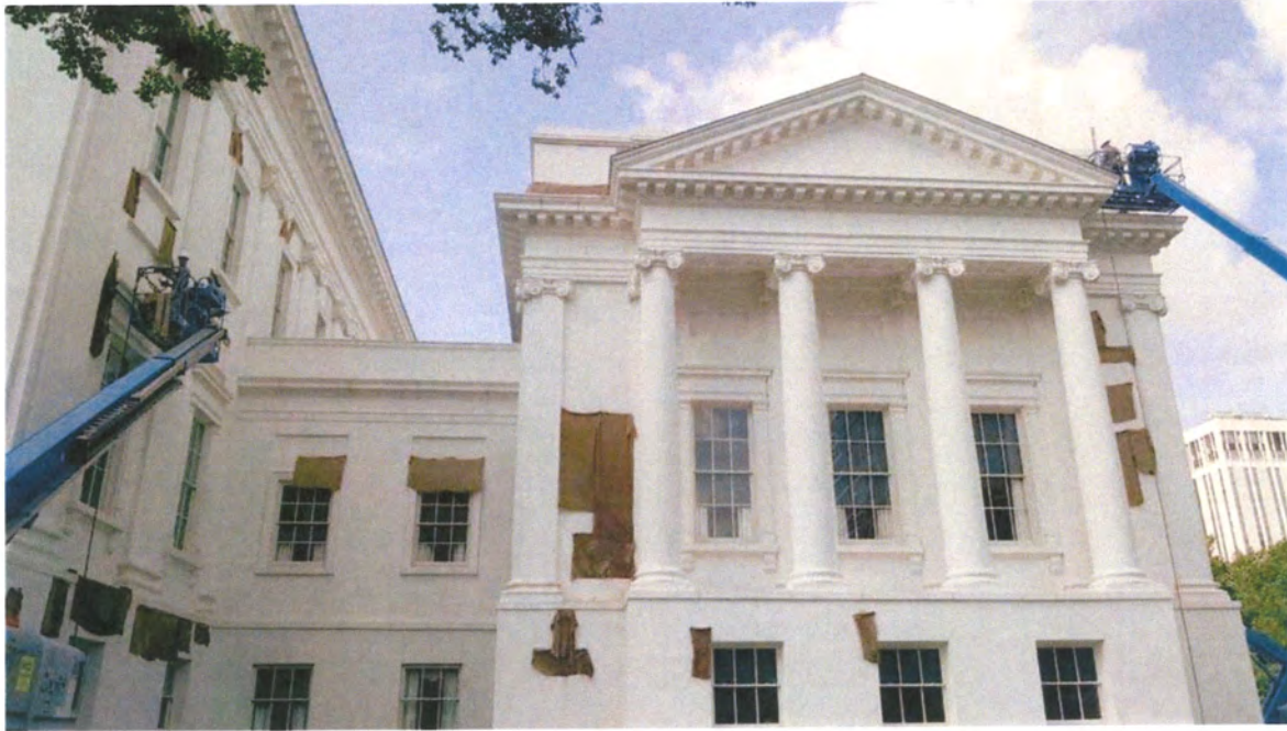
Figure 1: Virginia State Capitol Stucco Repairs covered in burlap to maintain moisture levels during curing period
