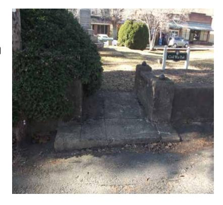
The intent is to eliminate the step and provide for an entrance with a running slope of maximum 8.33%.
