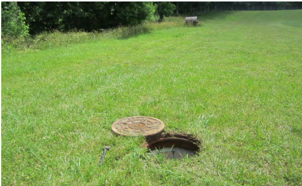
Photograph: Manhole installed at grade near forested area.
