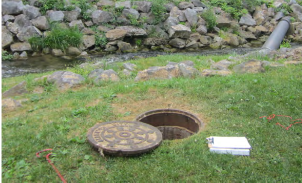
Photograph: Manhole at grade near small creek.
