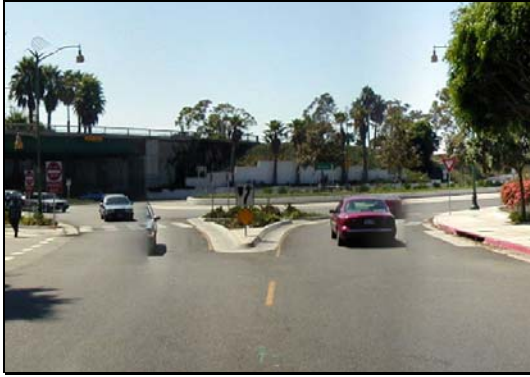
Median splitter islands and set-back crosswalks create safe pedestrian crossings
