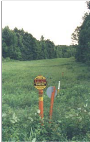
Gas pipeline corridor
