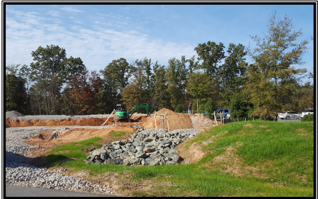
Image 4: A commercial building under construction at Zion Station
