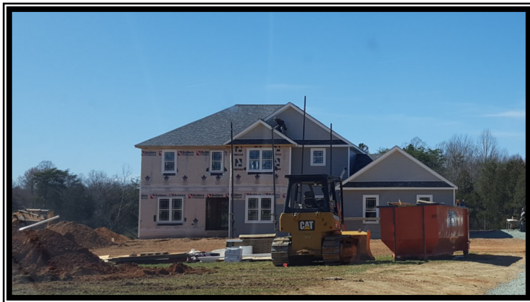
Image 6: A new house under construction
