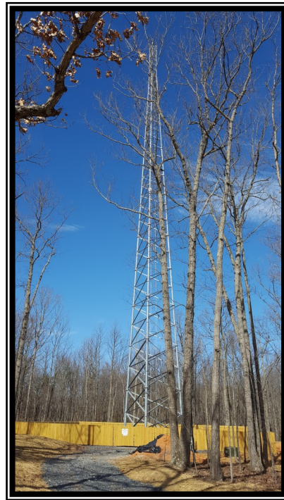
Image 9: Emergency Communications Radio Tower at a Veteran of Foreign Wars property (SUP 16:10)
