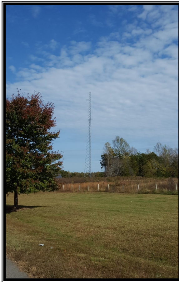
Image 8: Emergency Communications Radio Tower at the Sheriffs Office (SDP 16:04)
