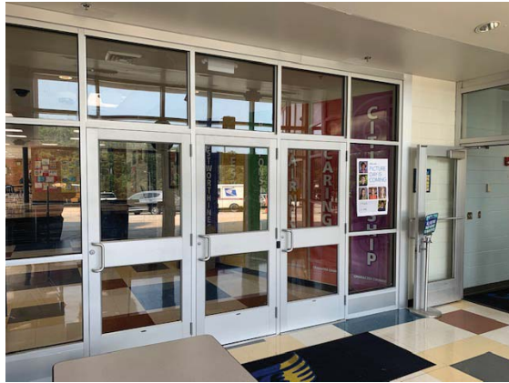
Central Elementary - Completed
