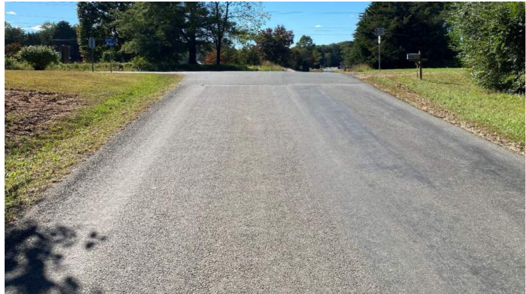
West along Route 697
