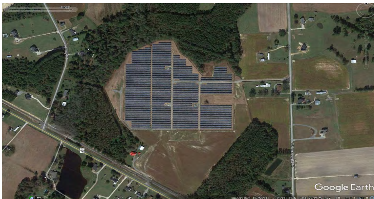
This 5 MW solar farm is located at 4839 US 70 Highway just east of Herring Road. This solar farm was completed on October 25, 2016.
