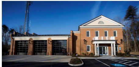
Figure 1, Palmyra Fire Company 1
