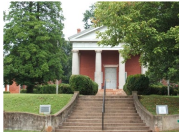
Figure LU-21, Historic Courthouse
