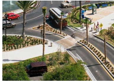
Figure LU-15, Median splitter islands and set-back crosswalks
