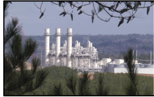
Figure NE14-8, Tenaska
