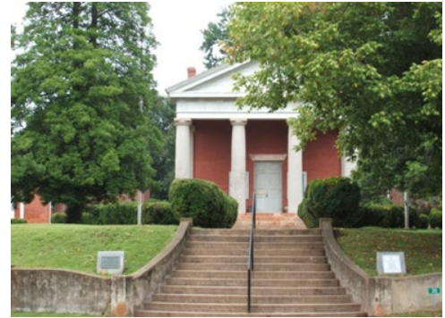
Figure LU-21, Historic Courthouse
