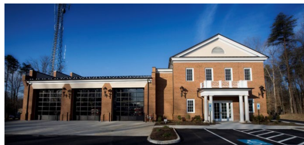
Figure 1, Palmyra Fire Company 1
